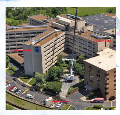
The most critical factor in choosing panels over sheet-metal ductwork was aesthetics. The panels and FläktGroup SEMCO's ability to customize, factory powder-coat, and color match them to the building's beige exterior actually appear as an accoutrement. Project architect FreemanWhite (Brentwood, TN) and consulting engineer TME (St. Louis, MO) paid strict attention to aesthetics, that the panels were factory designed, and assembled in sections where their seams matched the building seams.
