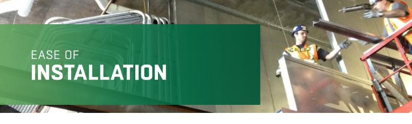
FläktGroup SEMCO assembly does not require screws at the panel joint. Our joint design will ensure a leakage rate of less than one half percent (<0.5%). This is achieved using only a bead of factory supplied LEED certified caulk. With no screws through panel joints, the possibility of air and noise leaks is eliminated and the installed cost is reduced.
