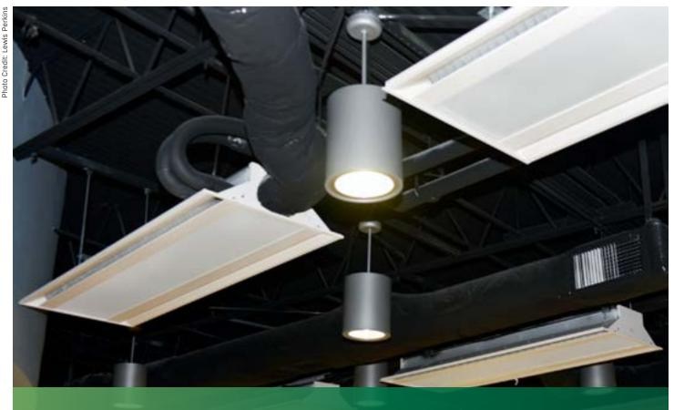
"We wanted to keep ceiling heights at 10 feet, so the inherent feature of the active chilled beams' reduced duct sizes caught our interest."
