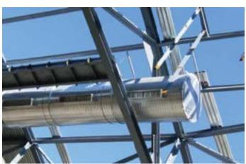
double-wall spiral duct as well as interior duct for the perimeter spaces of the arena. The manufacturer customized rectangular saddle taps to fit inside the round duct. These taps housed the large air diffusers required to direct air all the way to floor level of the arena. The
