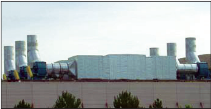
Exhaust Air Plenum
