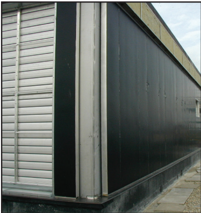
Louver Blank-Off Panels
