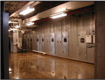
Built-Up Air Handlers
