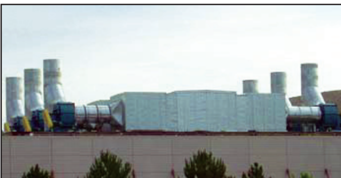
Exhaust Air Plenum
